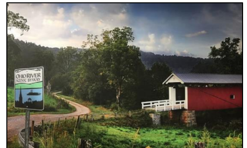
Figure 7. A covered bridge.
